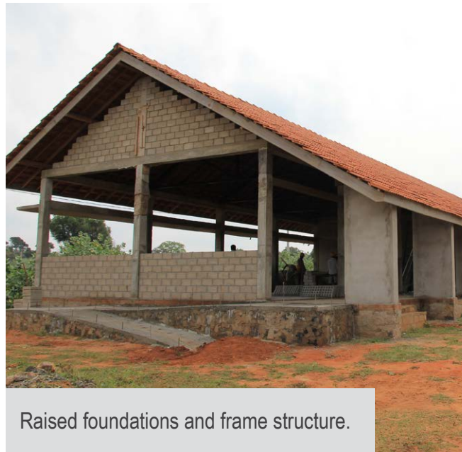
Tiled roof with a high roof gradient.
