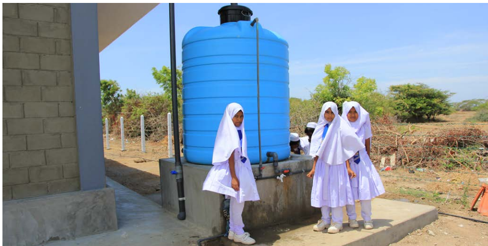
WASH facilities for girls at Periyapandivirichchan Primary School and RWH system and water tank at Koolankulam Government Muslim Mixed School.
