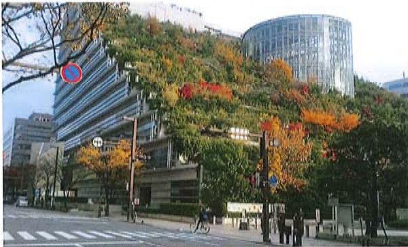
The ACROS building has 120 varieties of 50,000 plants, which keep the structure cool
