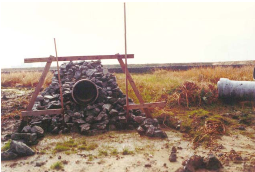
Imazu landfill – Images from period of landfill construction (1975 ~ 1999)
