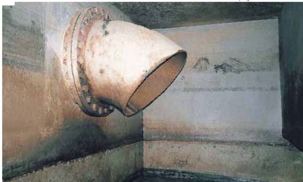
浸出水集排水管放流口 Collected leachate outlet pipe
