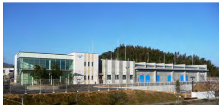
Hydrogen Energy Test & Research Center (HyTReC)
