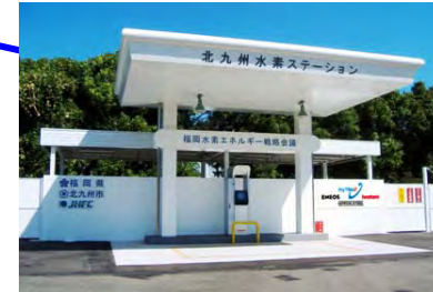
Hydrogen Station in Kitakyushu City (Based on by-product hydrogen supplied through a pipeline)
