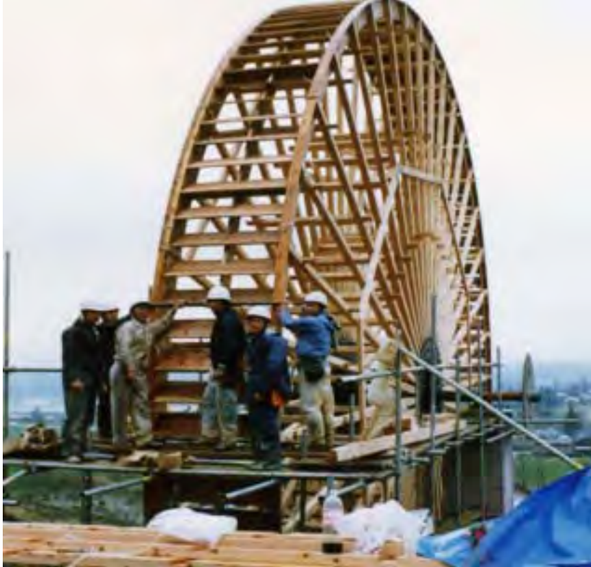
Overshot wheel for polishing rices. 14m in dia. Built in 1992
