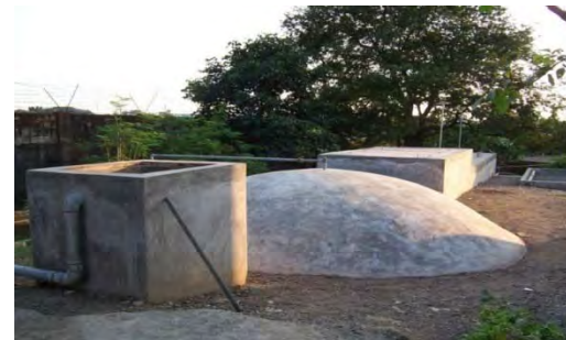
Valenzuela City Slaughterhouse Wastewater Treatment Facility with Biogas digester Model
