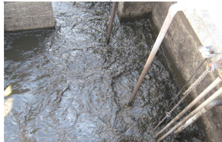
※Odor from the treatment tank was reduced, and the treatment capacity has improved. Also the odor was reduced in the aeration tank and removed scums.
