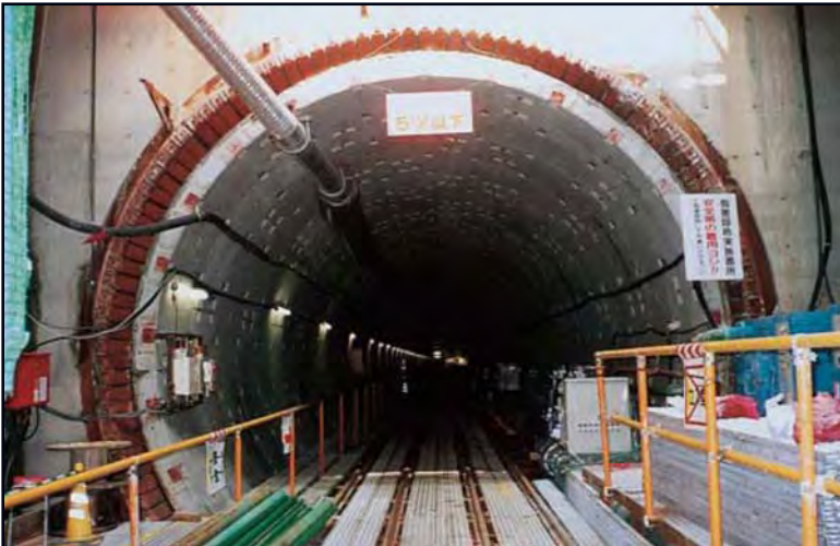
Maintenance of rainwater mains
