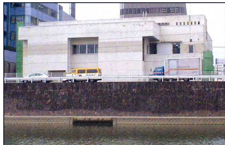
Maintenance of pumping stations
