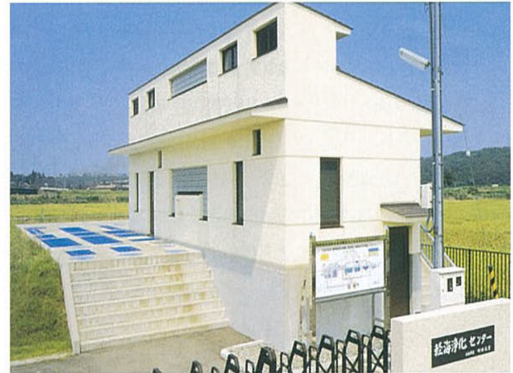
An RC-made johkasou for 740 NUD (JARUS type) (RC - reinforced concrete)
