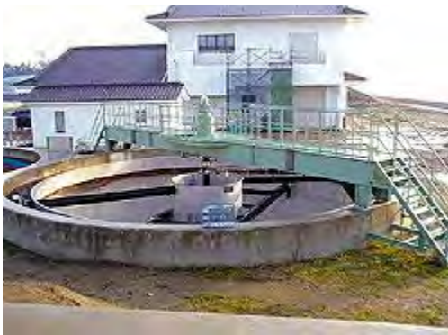
Sludge collector
