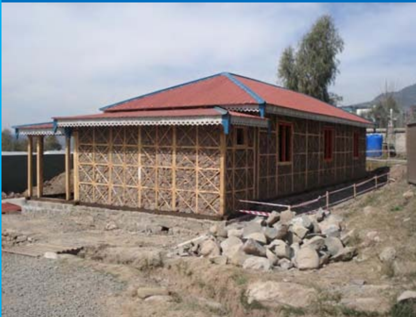
Timber frame stone infill (Dhajji)
