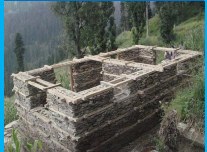
Timber reinforced dry stone masonry (Bhattar)
