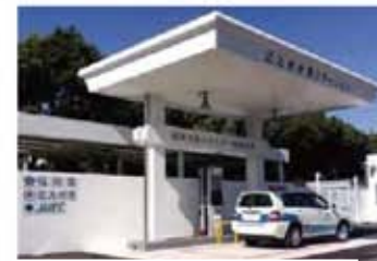
Kitakyushu hydrogen station
