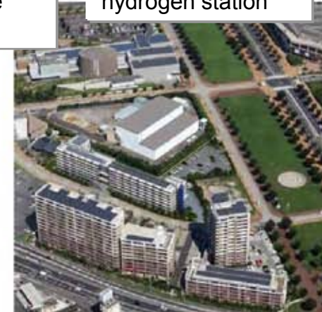
Photovoltaic generation panels installed on roofs of museum, company dormitory and condo in the Higashida street
