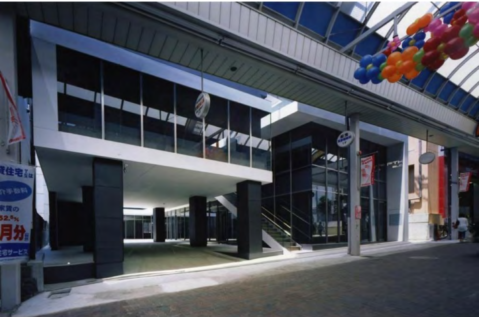
FTK Building after Refining
