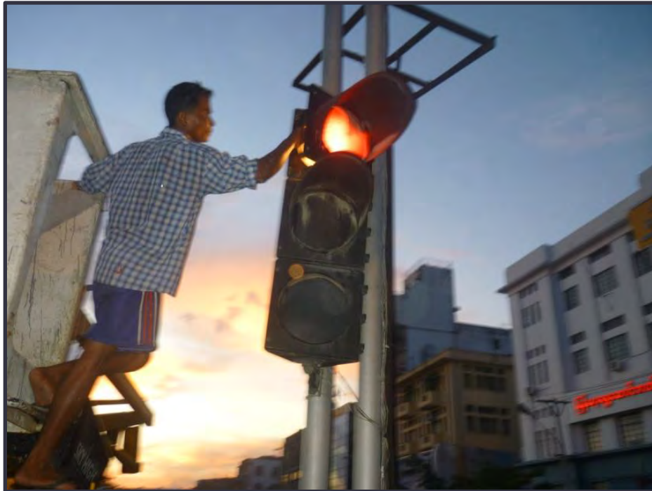
Upgrading of Junction Traffic Lights
