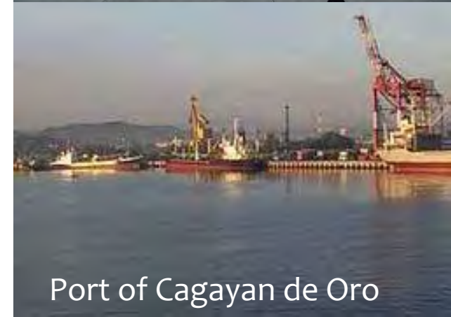
Mindanao Int'l. Container Terminal
