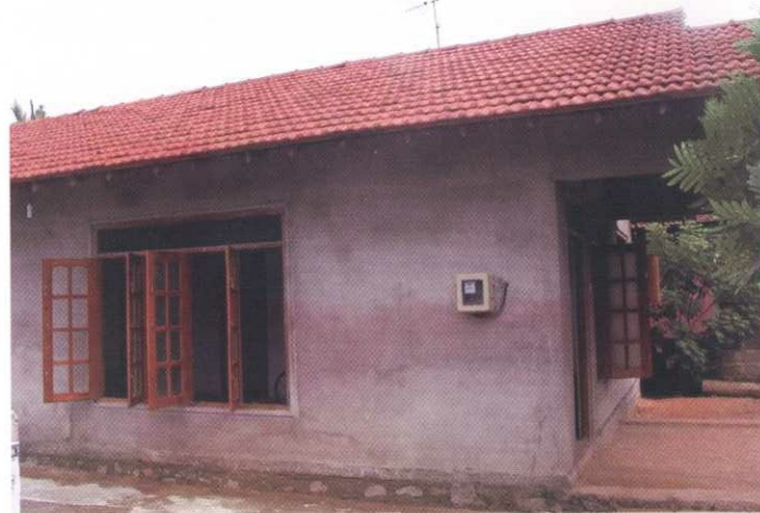
Completed House in Walauwatta, Galle.
