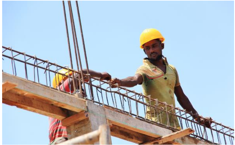
Construction work underway at Ikra Government Muslim Mixed School.
