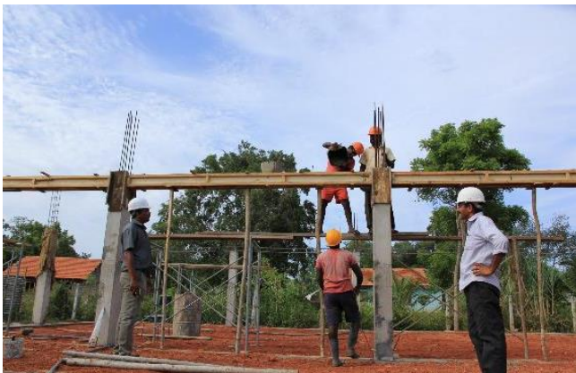
Construction work in progress at Periyapandivirichan Primary School
