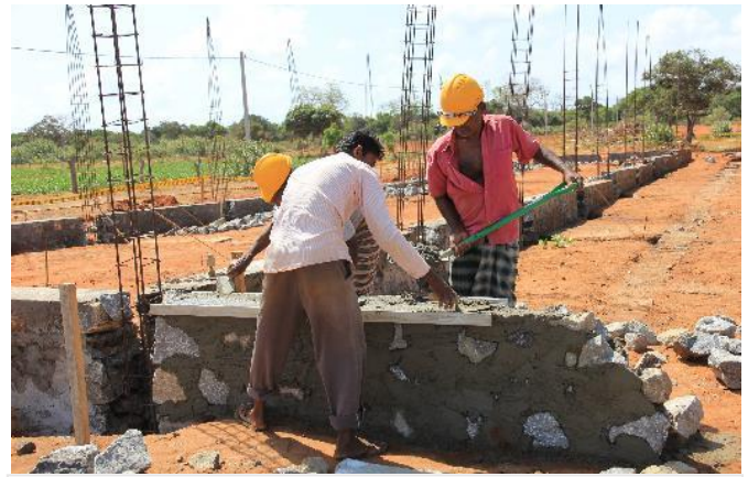
Foundation work in progress at Hunais Farook Government Muslim Mixed School.
