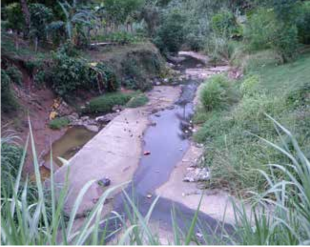
Poor drainage systems in Lautoka © SCOPE
