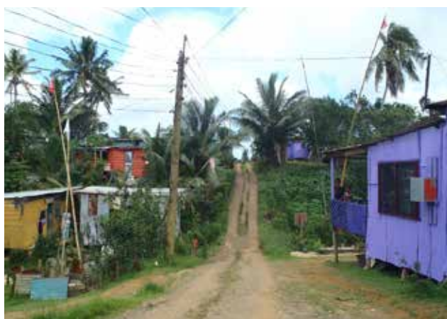
Power and telecom lines at Sasawira © SCOPE
