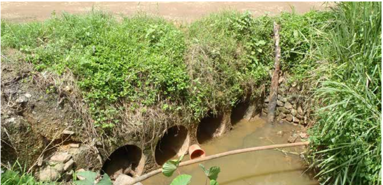
Roadside drains © SCOPE
