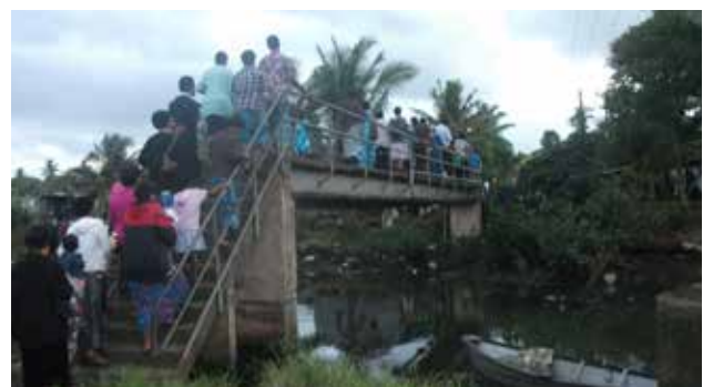
Pedestrian bridge access to Vatuwaqa settlement
