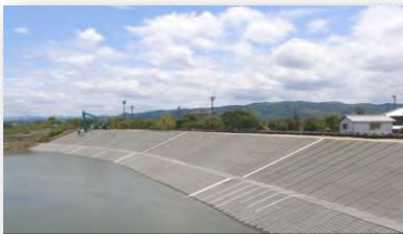
Fukuoka Prefecture (rehabilitated from the erosion damage)
