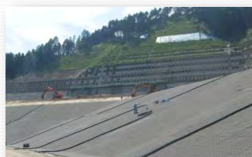
Saga Pref (embankment of dam river)
